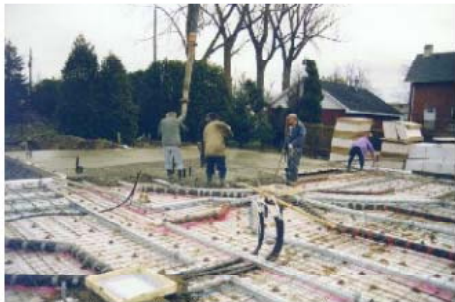
12. After inspection by LEGALETT installer, place concrete using vibrator.
