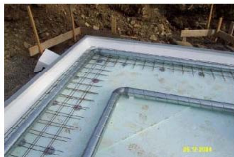
8. Cut and install piping
