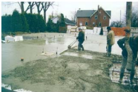
13. Steel trowel surface using power trowels. Hand trowel around furnace boxes.
