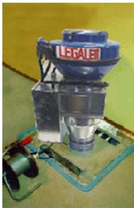
15. A LEGALETT construction heater can be used during and after placing the concrete and needs to be run for 2 weeks before flooring material installation or permanent insert installation
