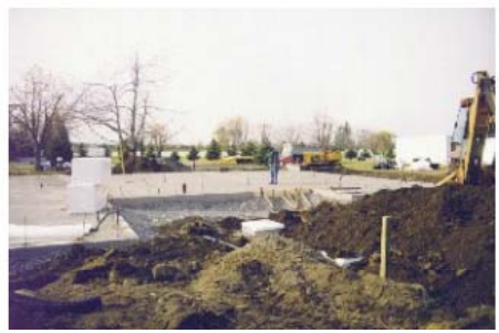
14. Keep top of slab moist for 3 days to minimize shrinkage cracking
