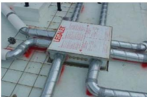
7. Install furnace boxes as per drawings and Product Data Sheets.
