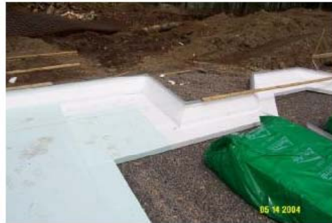
4. Install first layer of polystyrene insulation board.
