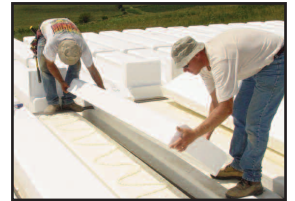
Foam glue is used to attach top-hats to the base section.
